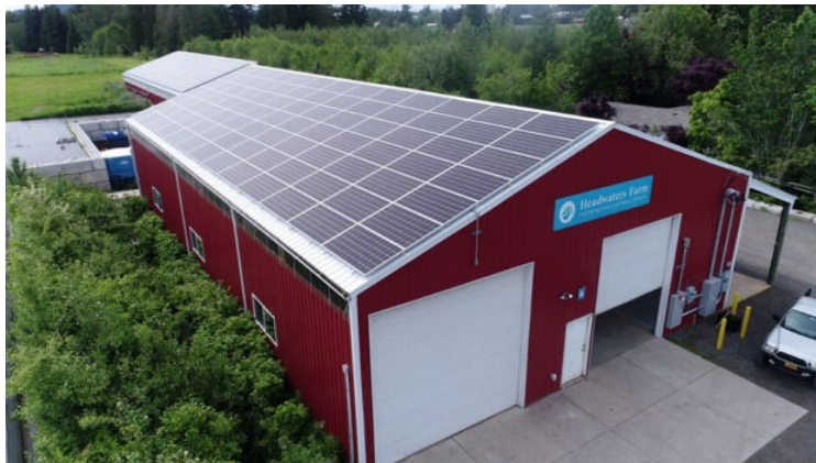
Solar panels atop the barn at the EMSWCD Incubator Farm
