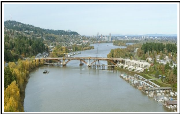
Completed in 2016, the new Sellwood Bridge has a steel deck arch design, adding to the city's unique bridge collection. It will withstand a major earthquake
