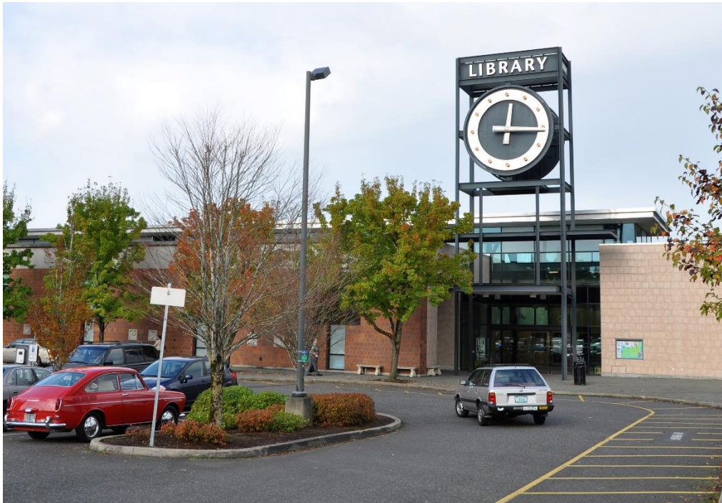
Figure 5: The Midland Library (on 122nd Street). TSCC used this facility for its annual budget law training this year.
