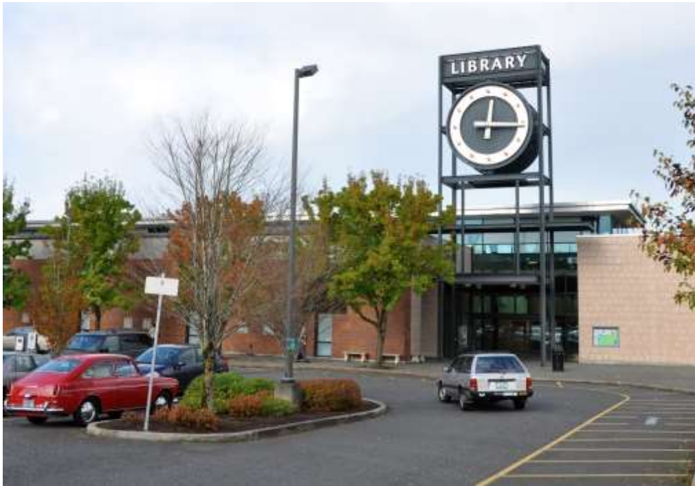
Figure 5: The Midland Library (on 122nd Street). TSCC used this facility for its annual budget law training this year.
